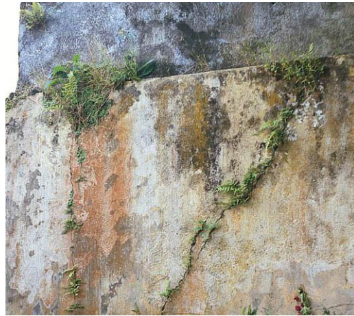
Image 28. Weathered white-washed stucco
